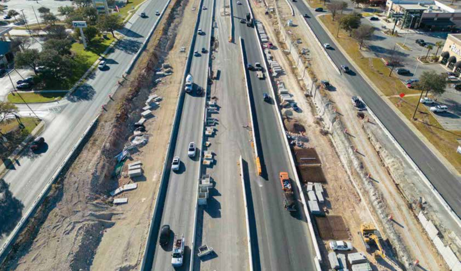
Fig. 6: Roadway repair project 9
